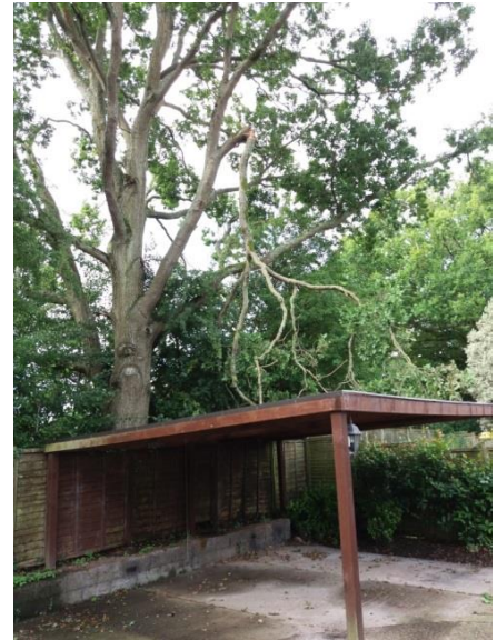
Failed oak limb hanging over a car port in North Baddesley
